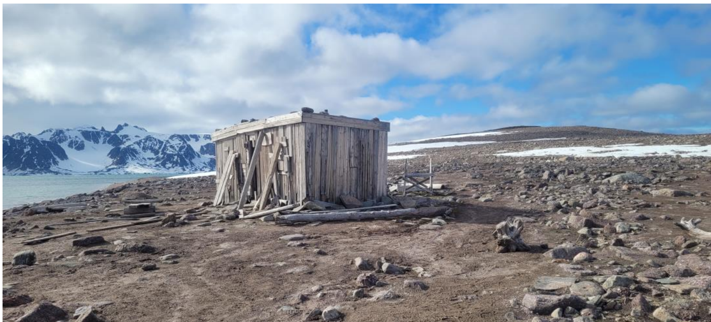
Old trapping hut on Alicehamna.
